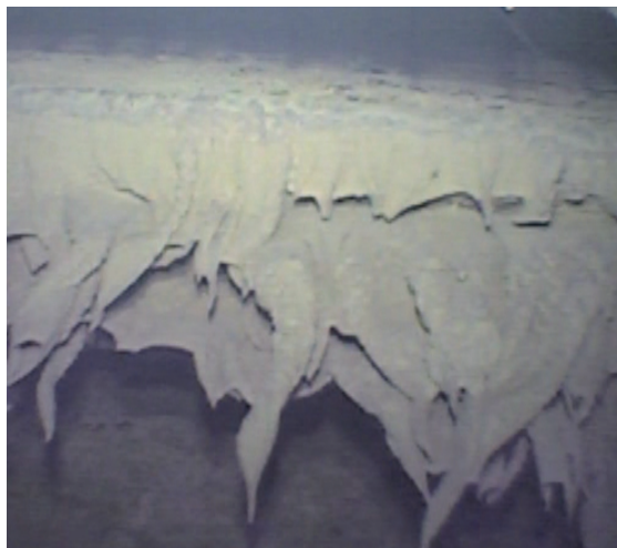
Substantial build up of deposits on an Economiser installed in a Waste To Energy plant
