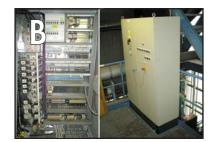
A plc based monitor and control system enables unmanned automatic operation which is relayed to the regular control room for alarm and monitor functions.
