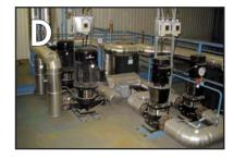
The cooling water system which enables the Ecotubes to operate continuously within the furnace comprises a pump, a heat exchanger and auxiliary equipment. Extracted energy can be utilised for various purposes within the plant energy system.
