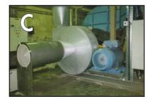
A dedicated high pressure process air system comprising skid mounted fan, ductwork and adjustable Ecotube distributed nozzles provides the increased flue gas turbulence and mixing within the furnace.
